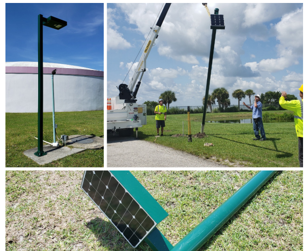
City staff converting outdoor lighting to solar-powered lighting
