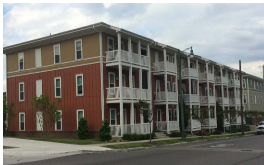
South Junction, the first development to participate in MLGW's Energy Advantage Apartments program.
