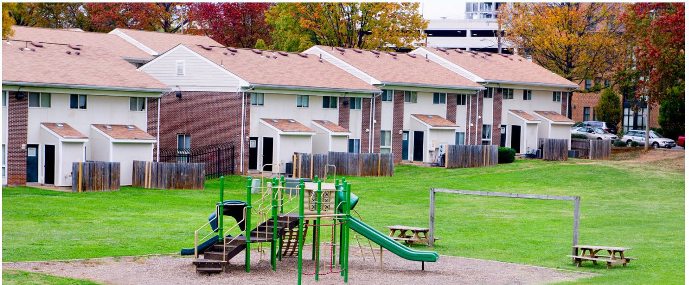
Friendship Court, Charlottesville, Virginia. NHT-Enterprise invested over $250,000 in high-efficiency HVAC systems, appliances, and lighting, reducing annual operating costs by $50,000.
