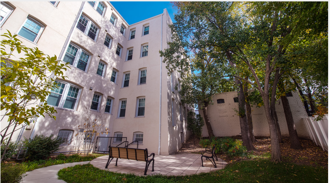
St. Dennis Apartments, Washington, D.C. NHT-Enterprise upgraded this property including energy efficient heat pumps, hot water heaters, and Energy Star appliances to meet Enterprise Green Communities Criteria while also maintaining important historic features.
