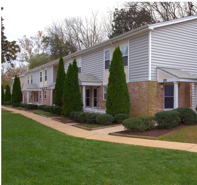
Hazel Hill Apartments, Fredericksburg, Virginia.
